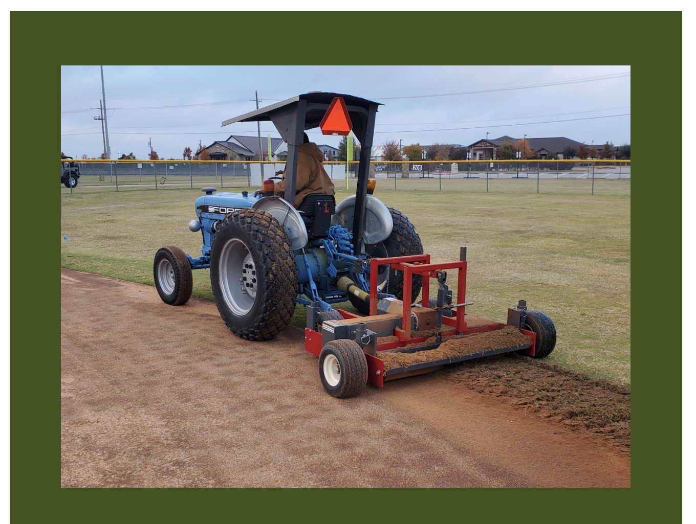
LEON TUTTLE ATHLETIC COMPLEX RENOVATIONS HAVE BEGUN
